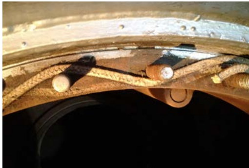
Joint tresse amianté
